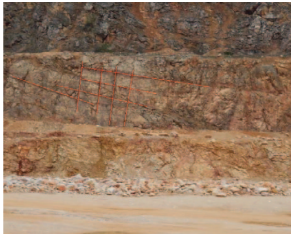
Figure 4. Drilling conditions and limestone discontinuity on limestone quarry "Vijenac"
