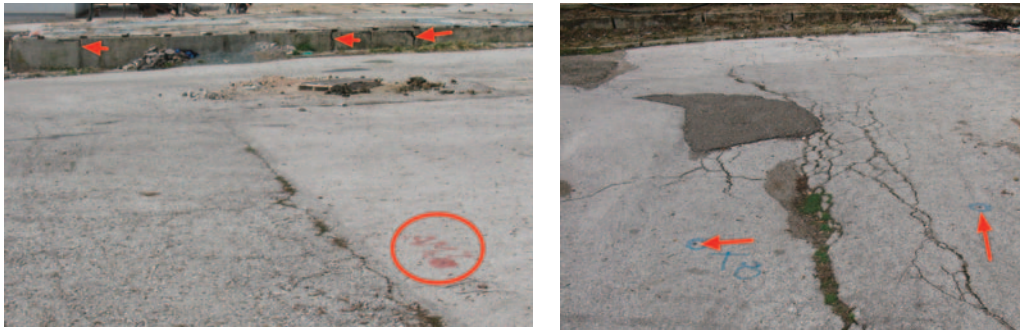
Figure 4. Left: Polygon point AM3 with the route of the scar perpendicular to the destroyed object “Amos”. Pronounced deformations (orientation and slope of the fracture in the southern direction) on the foundation wall. Right: Display of the built-in benchmark. “Settling scars” in the form of cracks in the asphalt with clearly expressed elements: the width of the impact and the direction of stretching. (Photo by J. Čomić).
