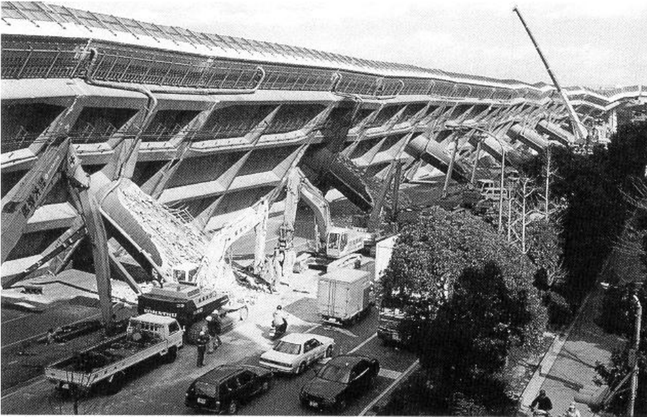
TYPICAL BRIDGE COLLAPSE: B) NORTRIGE, U.S.A., 1994, M=6.7: PIER'S TOTAL SHEAR FAILURE
